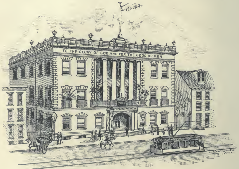
ASSOCIATION BUILDING, MAUCH CHUNK, PA.
